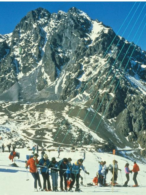
The infamous Roca Jack lift in Portillo, Chile. The "Va et Vient" is a strange invention which has five Poma lifts all connected together - without any lift towers.
