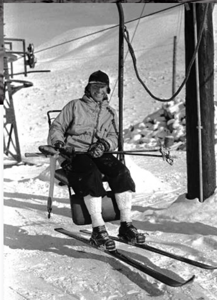
The world's first chairlift, installed on Dollar Mountain, was based on banana hoisting equipment used on cargo ships of this era.
